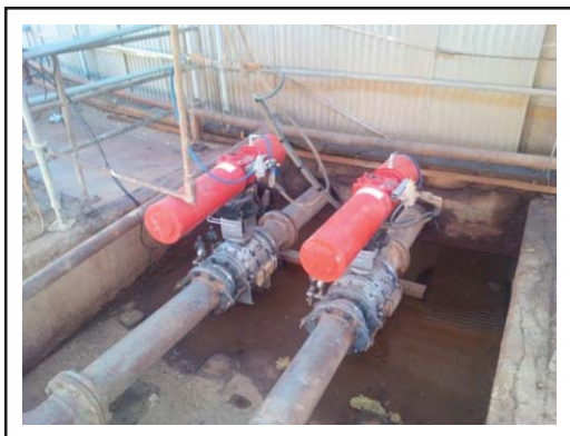
Quad-Master® with Ring Master® Seating System for Geothermal Brine Clarifier Tank Valve
